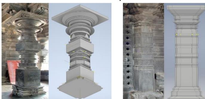
Fig.3. Columns with developed three-dimensional models
